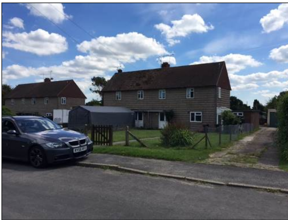
Figure 2 – Existing external finishes
